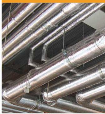
Mineral Wool (Stone & Glass) products have been the mainstay for warm and hot services in HVAC installations for many years. This tried and tested type of insulant offers additional performance characteristics such as fire resistance and acoustic absorption and is often the first choice in value engineered solutions. The different forms are easy to cut, fit and maintain, making them one of the first choices for insulation contractors.
