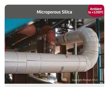
An insulation material with very good thermal properties for higher temperature applications.
